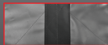
Patch over seam
